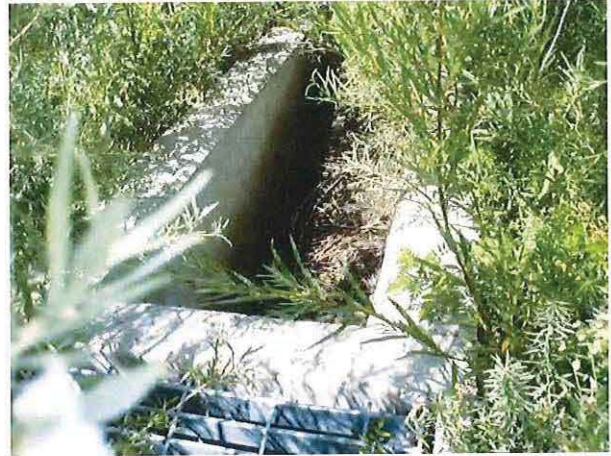
Photo 35 – WBR Outlet Structure
