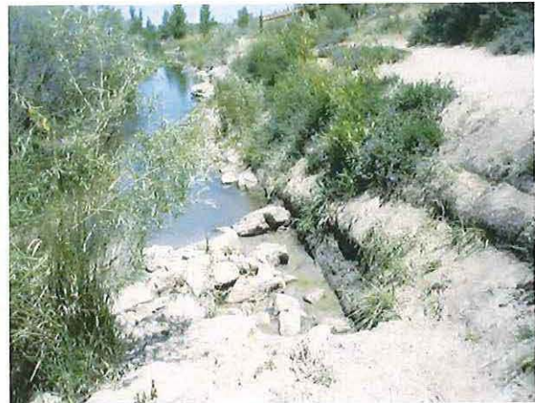
Photo 17 – 12-Mile Park, Phase II, Soil Wrap Bank Stabilized Area
