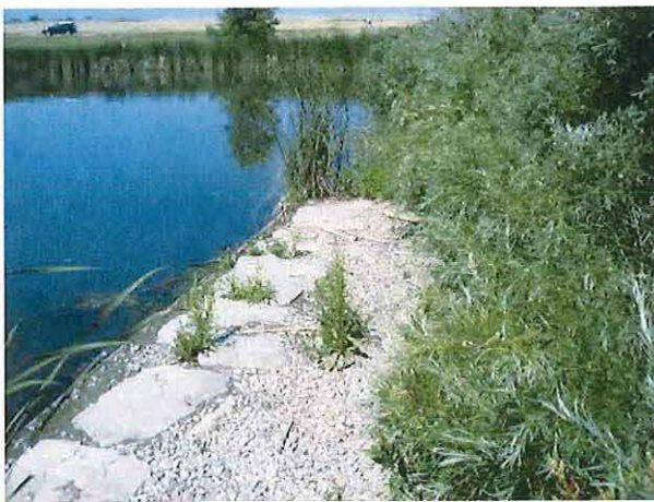
Photo 10 – Cottonwood Wetland Shoreline Stabilization
