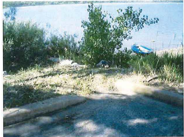
Photo 25 – East Boat Ramp Curb Cut Drainage
