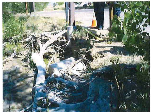
Photo 23 - East Boat Ramp Shoreline Erosion
