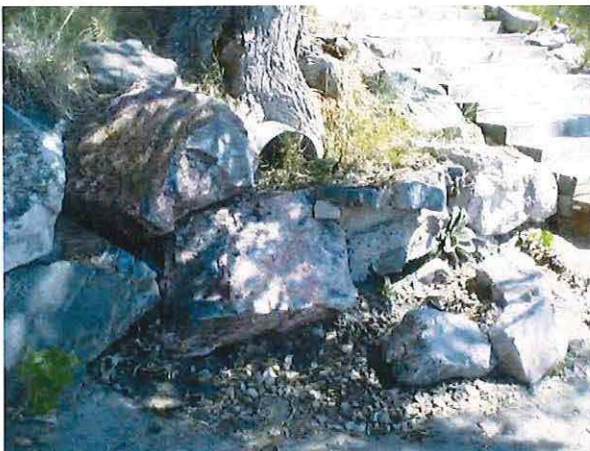
Photo 29 - Tower Loop Parking Lot Drainage Outfall
