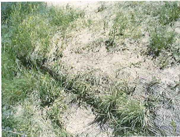
Photo 18 – 12-Mile Park, Phase II, Soil Wrap Bank Stabilized Area
