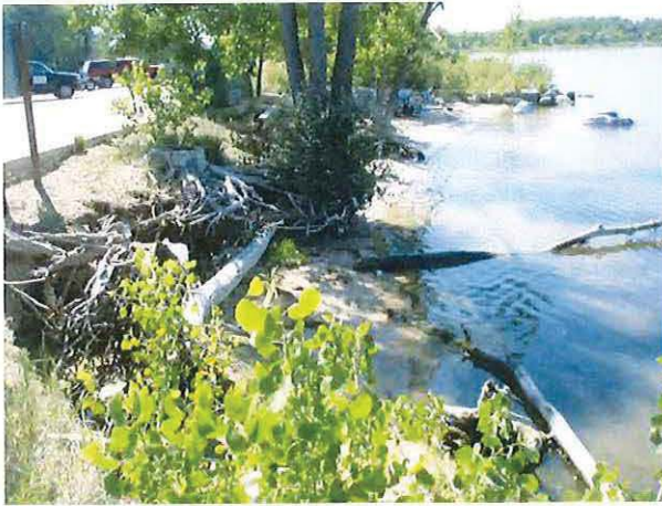
Photo 24 – East Boat Ramp Shoreline Erosion
